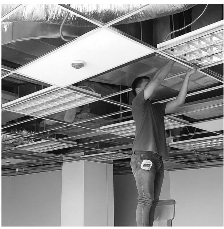
In this image, the worker is installing or adjusting acoustical ceiling tiles but is standing on an unstable chair instead of a proper ladder or scaffold. This practice significantly increases the risk of falling and injury. There is also no visible personal protective equipment (PPE) such as gloves, safety glasses, or a helmet, which would be essential in case of falling debris or accidental contact with sharp edges or exposed ductwork.
