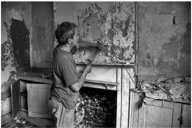
Look at the image above, there is a man working around a huge quantity of asbestos, he probably does not know much about how bad asbestos can be. He is working without any personal protective equipment; he should be wearing a respiratory protection at least.
