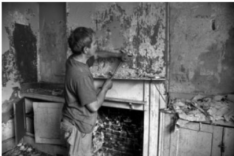
Look at the image above. There is a man working around a huge quantity of asbestos and he probably does not know much about how bad asbestos can be. He is working without any personal protective equipment; he should be wearing respiratory protection at the very least.
