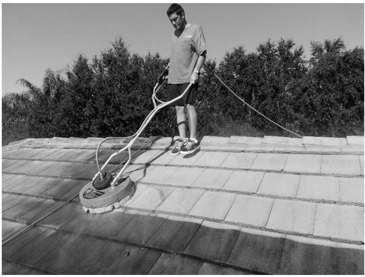
The image shows a worker pressure washing a sloped roof without any visible fall protection or proper safety gear. He is wearing sneakers, which lack the necessary grip for working on wet surfaces, significantly increasing the risk of slipping. Additionally, the long hoses and cables are spread out across the work area, creating a serious tripping hazard. The lack of proper control over the equipment and footing on a wet surface further increases the likelihood of an accident.
