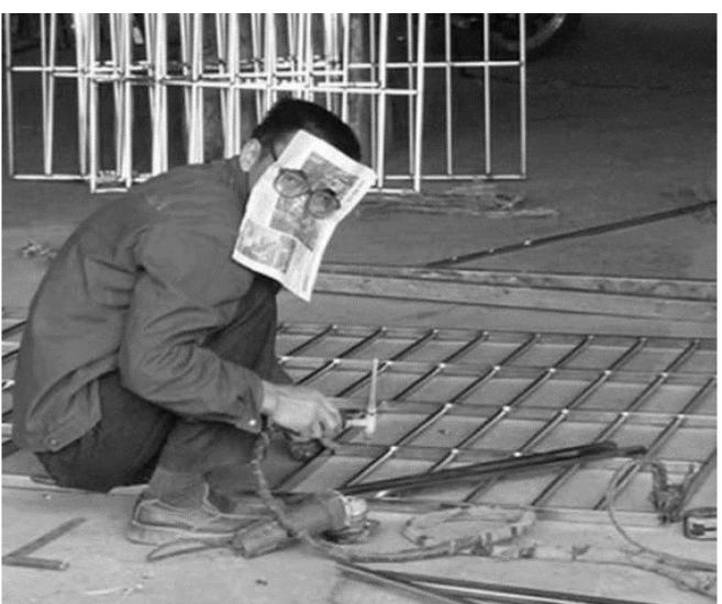
What is wrong in this picture? There is a guy working on welding with any proper PPE. He is using a paper to protect his face from carbon monoxide exposure.
