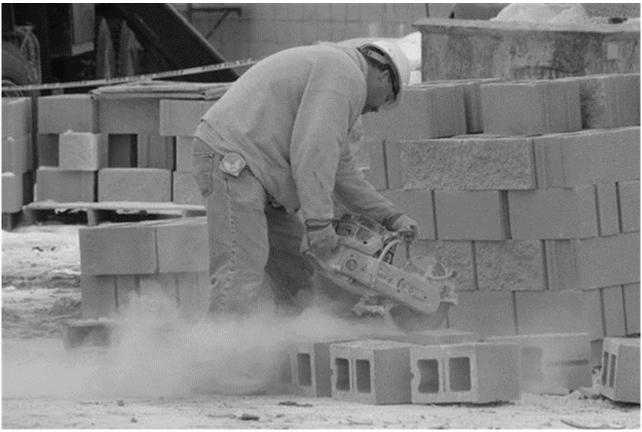
Look at the image above and see what is wrong in the picture, there is a construction worker doing a task around a high exposure of dust without any proper PPE. Construction workers have been identified in many other studies as being at risk of exposure to a number of carcinogens, particularly asbestos, wood, dust, crystalline silica, solar UV radiation and diesel engine exhaust.
