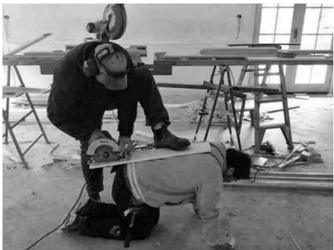
In this image, workers are using power tools in a highly unsafe and improvised setup, with one person acting as a sawhorse and no apparent fall, eye, or hand protection in place. This scenario shows the dangers of ignoring proper PPE and safe practices in carpentry. When workers cut corners on safety, they risk severe injuries from saw blades, falling objects, or flying debris.
