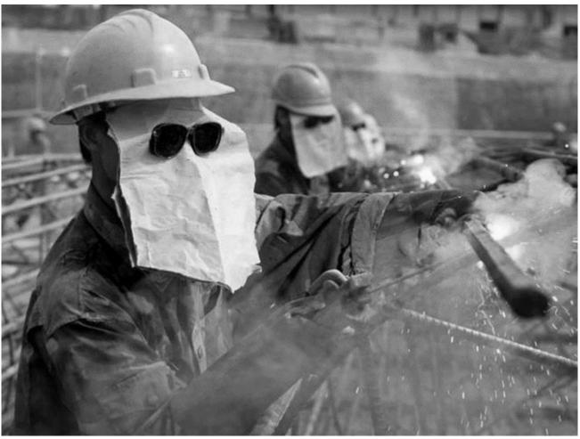
What is wrong in this picture? There are a group of construction worker who are not wearing proper welding helmet instead of that they are using a piece of cement sheath to protect their face.
