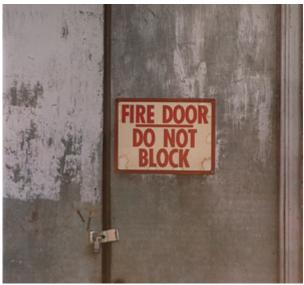
Imagine that you were a worker inside this building counting on getting through that exit to flee a fire. That padlock is sealing not just your escape exit but your fate.
