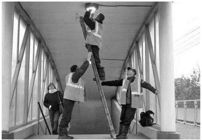
What's wrong in this picture? There are a group electricians working inadequately on a ladder, they are putting their co-worker in danger because of the unsafe procedure that they are doing to do the task.
