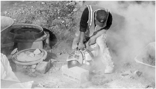
What's wrong in this picture? There is a construction worker who is working around excessive dust and he is not wearing any proper PPE to avoid dust hazards.
