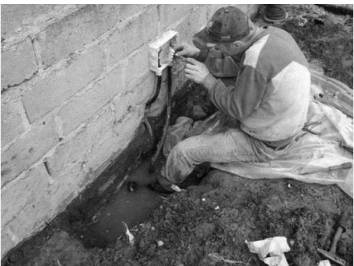
What's wrong in this picture? There is a worker who is into contact with an exposed electric conductor or part of a circuit and his feet are under the water. This can cause heart problems, muscle spasms, and loss of breath. This type of injury is more serious and can often end in death.
