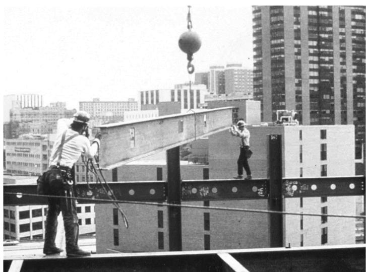
What's wrong in this picture? there are two workers working at heights and have any kind of fall protections. Falls are among the most common causes of serious work-related injuries and deaths. If a fall hazard cannot be eliminated, effective fall protection shall be planned, implemented, and monitored to control the risks of injury due to falling.
