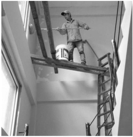
What's wrong in this picture? There is a man painting a wall without any fall protection. He is standing on thin boards that are not well secured. How dangerous and painful can it be if this person falls from that height?
