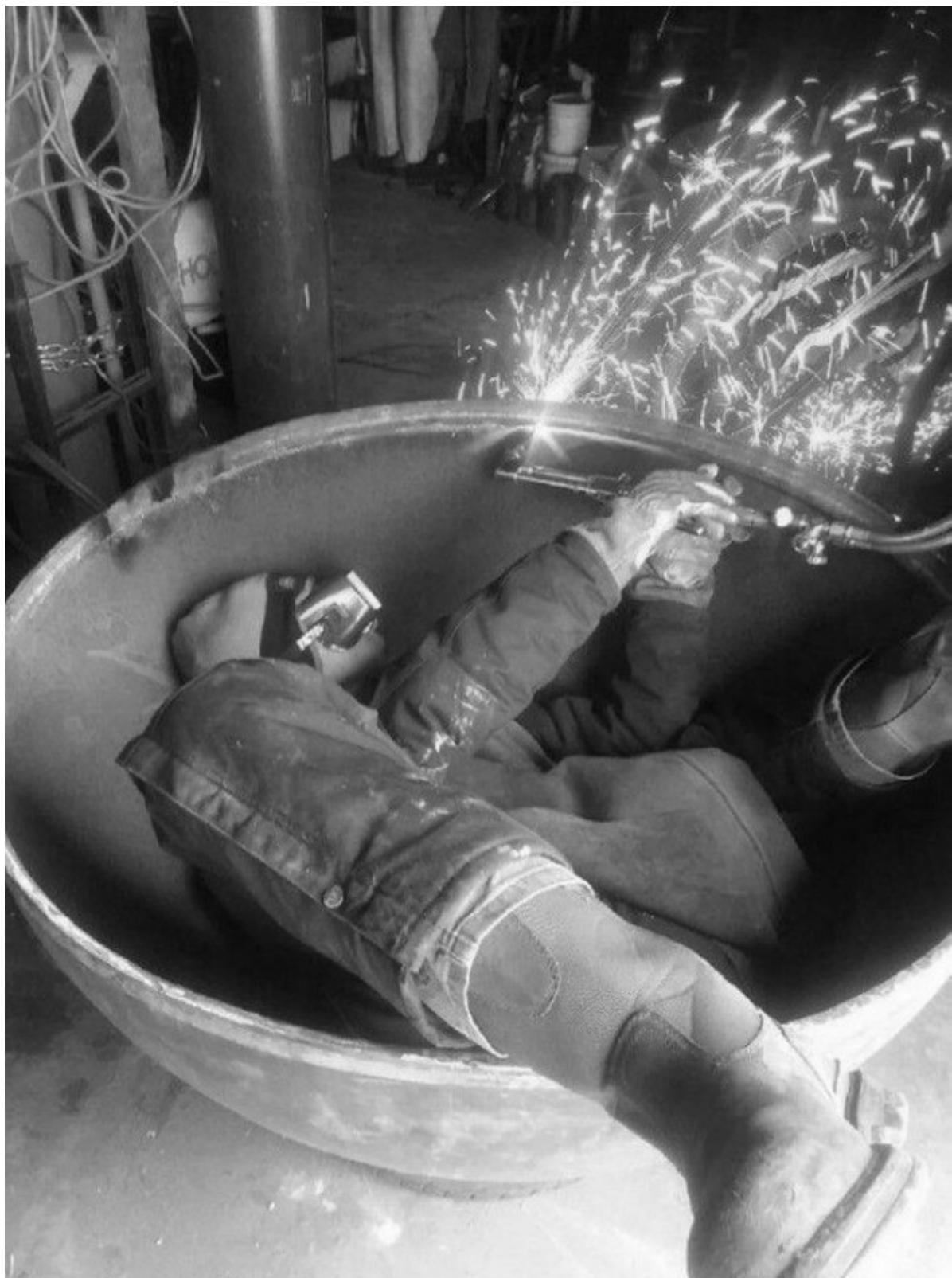
Hot work can throw sparks and molten material more than 35 feet during welding, cutting, and grinding. These sparks and hot slag are typically burning above 1,000°F—more than enough to easily ignite paper, wood, flammable liquids, vapors, and any other combustibles in the area.
