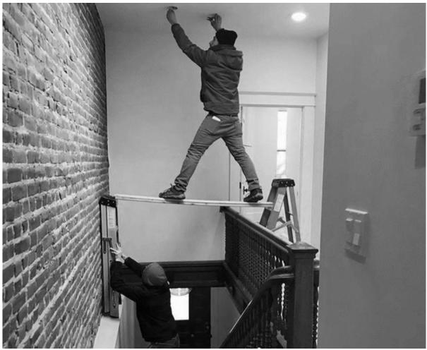
What's wrong in this picture? There is a worker trying to put a spotlight on the wall but he is not paying the necessary attention to how he is doing it, he is not wearing any fall protection and the walking space on the plank is limited and awkward which makes any movement dangerous.
