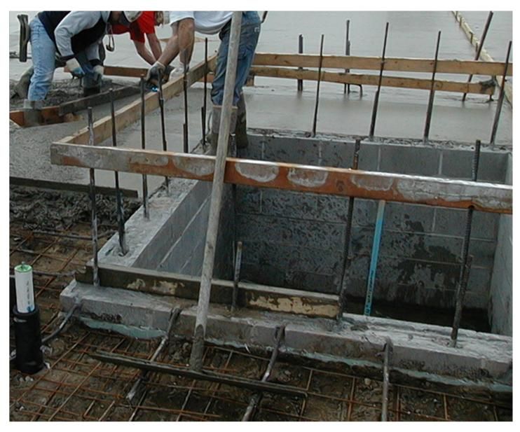
The railing arrangement in this photo is in some ways more dangerous than the floor hole it's guarding:
