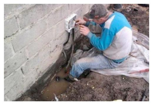
You don't have to be an electrical engineer to recognize that it's not a great idea to repair electrical equipment with one's feet immersed in a puddle. It's just too bad the gentleman in the photo didn't get the memo.
