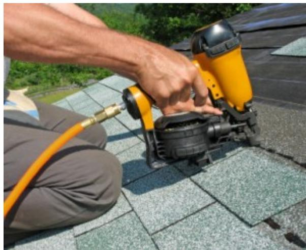
**2. Contact Triggers** which fire a nail when the safety contact and trigger are activated in *any* order.
