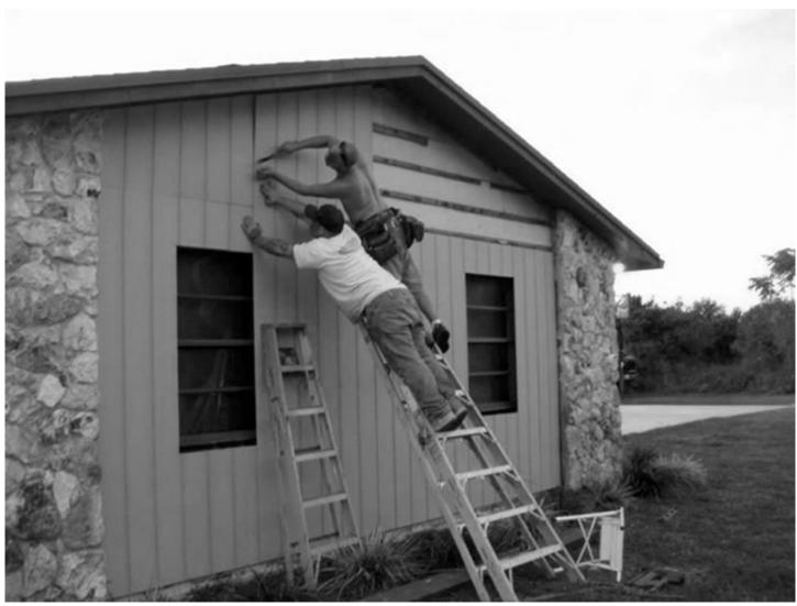
This image demonstrates a highly unsafe ladder use scenario. One worker is standing on top of a closed step ladder that is not fully opened or locked, while another person is dangerously climbing over him. Additionally, a second ladder nearby is not being used but is also positioned unsafely. These behaviors violate basic ladder safety rules and present a high risk of falls and serious injury.
