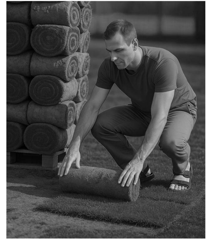
The worker in the image is laying down sod without using proper personal protective equipment (PPE). He is wearing open-toe sandals, which offer no protection against heavy or sharp objects like tools, rolls of sod, or sharp debris hidden in the grass. His hands are unprotected as well—without gloves, he is at risk for cuts, blisters, and exposure to soil-borne bacteria or chemicals. Additionally, no knee protection is used despite prolonged kneeling.
