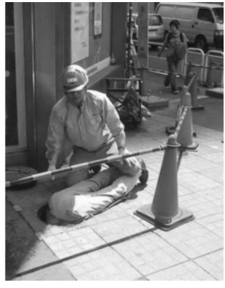
If the worker is "distracted" or interrupted by someone coming out of the door or by a passer-by pedestrian, the worker he is holding down is a dead man!!
