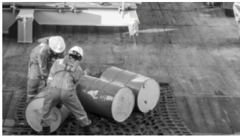
Worker NO.1. is in danger of having his right foot being "rolled up" by a large drum by employing unsafe handling technique/procedure. Solution: The drums should have been separated by the workers.
