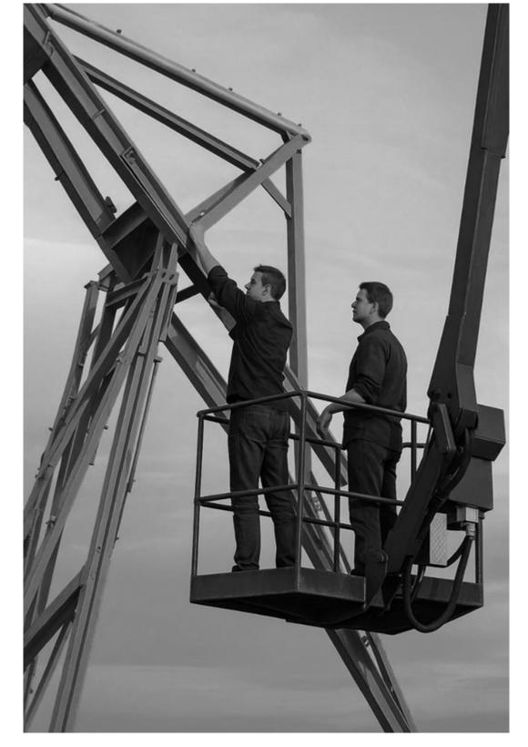
This image shows two workers on a mobile elevated work platform (MEWP), but several safety concerns are visible. Neither worker is wearing a safety harness or fall arrest system, which is essential when working at height on MEWPs. Additionally, they appear to be standing very close to the edge without proper anchorage or protection.
