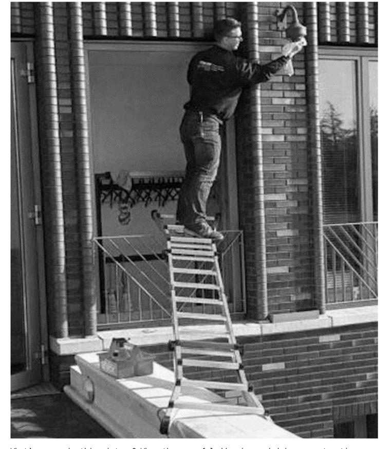
What's wrong in this picture? When the use of ladder is needed in a construction site, be sure you must be conscious in how, and where you are setting up your ladder to do your job, which is missing on the picture above. The lack of safety practices can result in an injury or even in a fatality.
