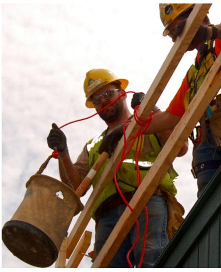
Picture This nearly always focuses on unsafe work practices, but this week we have a photograph showing workers doing the right thing. In this case, a worker is shown using a bucket and rope to hoist tools to an elevated work area. This arrangement allows workers to maintain three points of contact when ascending or descending ladders. (eLCOSH)
