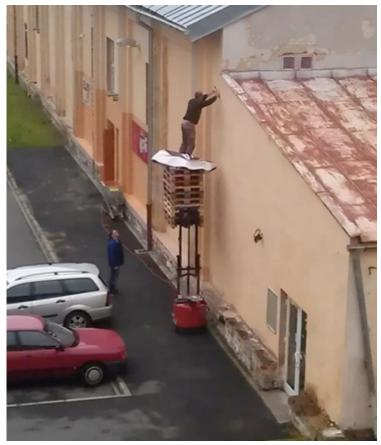
There is a right way and a wrong way to do things. Guess which method is illustrated here? A worker risks life and limb by standing on a stack of pallets piled on top of an aerial lift. To make matters worse, he is leaning forward to reach the wall, all without using any form of fall protection. (Fail Blog)
