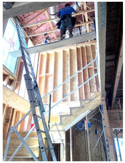
Ingenuity at its finest or accident waiting to happen? The walking space on the plank is limited and awkward which makes any movement dangerous. Reach back for the hammer, lose balance, slam into the stair guardrails on the way to concrete floor below.
