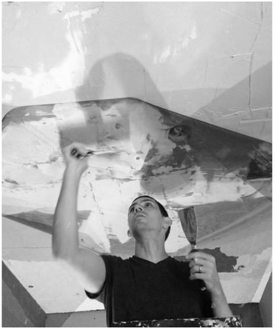
In this image, the individual is plastering a ceiling without appropriate protective equipment. This poses several risks: debris or wet plaster could fall into the worker's eyes, and extended overhead work can strain the neck, shoulders, and arms. Additionally, if the worker is standing on an unstable platform or lacks proper footwear, falls or slips could occur.
