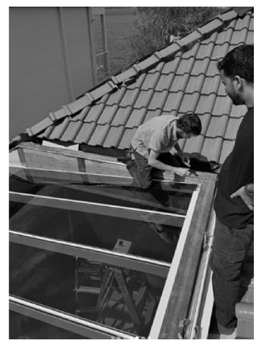
The image shows two workers on a sloped roof near a large glass skylight, with one actively working on the structure. There are significant safety hazards present, as neither worker appears to be using fall protection equipment, such as a harness or an anchored lifeline. Additionally, the worker is positioned directly above the skylight
