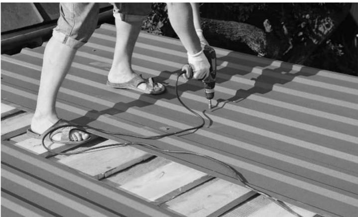
In the image, a person is standing on a metal roof while using a power drill. However, they are wearing open-toed sandals, standing on an unstable surface without visible fall protection, and handling electrical equipment with exposed wiring. This situation presents multiple serious hazards, including fall risks, electrocution, and foot injuries from tools or materials.
