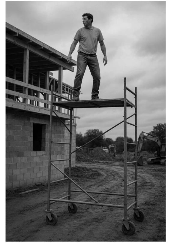
This image highlights a major scaffold tower safety issue. The individual is standing on a scaffold platform without any guardrails, fall protection, or visible stabilization. Additionally, the scaffold has wheels and appears to be unsecured, which increases the risk of movement and collapse. Working at height without proper precautions puts workers at serious risk of injury or death due to falls.
