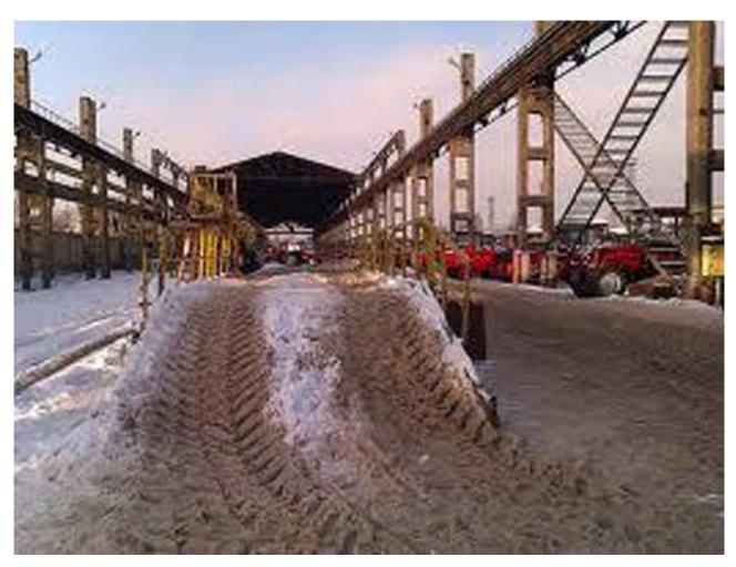
A hazard even in perfect weather conditions, ramps like the one in this picture become an even greater slip-and-fall danger when they're covered in snow and ice. Although it appears that the ramp might have been sanded, it would have been a lot safer had the snow and ice been completely removed.
