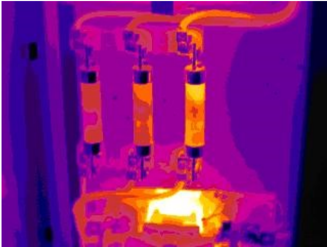
Iron palette of fuse bus bar
