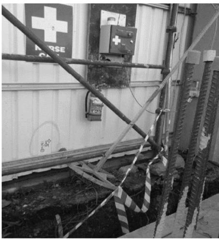
Look at all the obstructions in the way of this fire extinguisher—crossed rebars, safety tape, mounted cables and an open trench. All that's missing are alligators in the moat!
