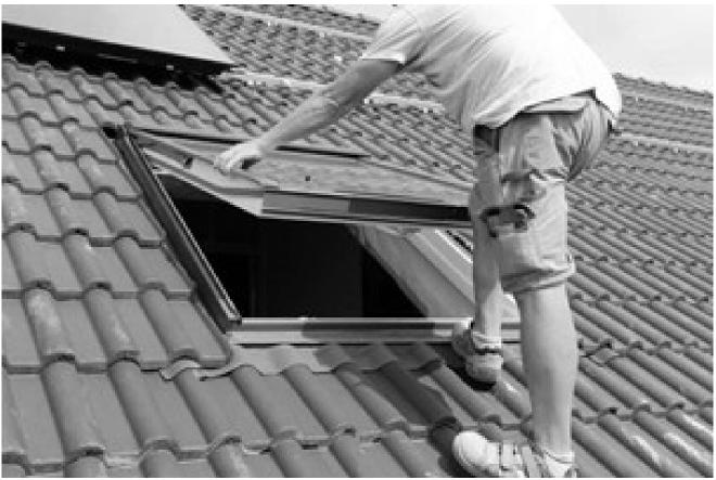
The image shows a worker handling a skylight on a sloped roof without visible fall protection. The individual appears to be wearing standard sneakers rather than proper slip-resistant footwear designed for roof work. Additionally, there are no safety harnesses, guardrails, or other fall protection measures in place, which are crucial when working at heights. The risk of falling through the skylight or off the roof is high, which could result in severe injuries or fatalities.
